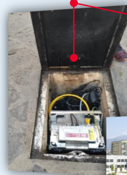
Sorrento small cell in a manhole
